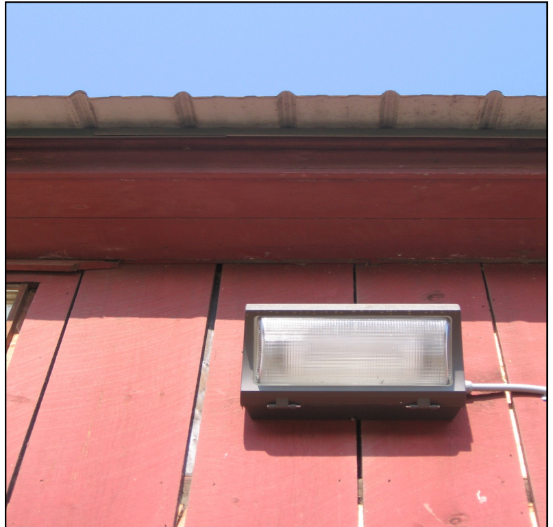
An outdoor metal halide fixture can save as much as $160 per year.
