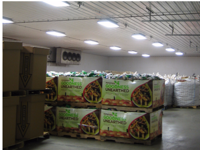
LED Lighting upgrade at Szawlowski Potato Farm, Hatfield.
