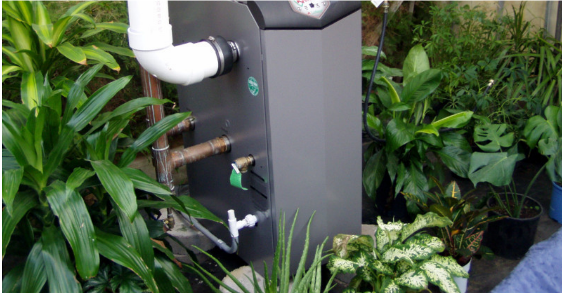
Example of an energy efficient heating system at work in a greenhouse
