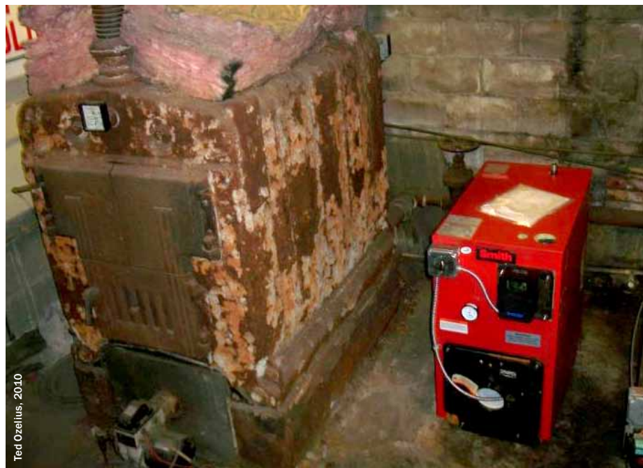
Dutchie's Greenhouses, in Plymouth, MA, replaced their old boiler (left) with a new, efficient boiler (right).
