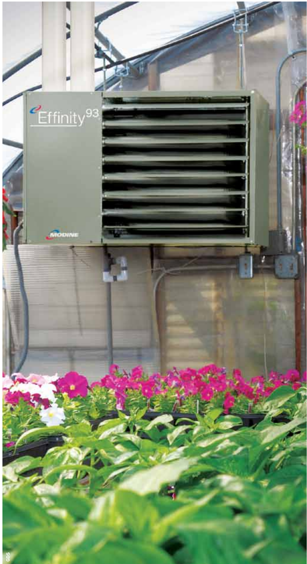
New gas-fired unit heaters are rated to operate at 93% efficiency.
