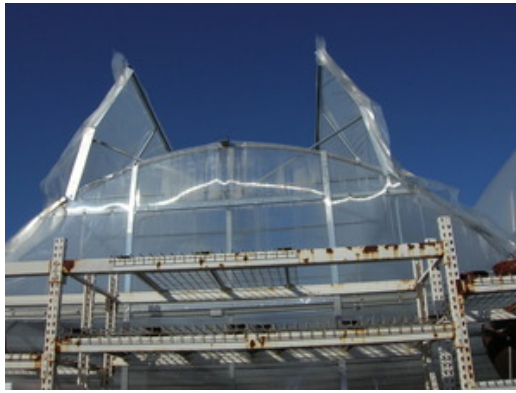
Greenhouse with passive roof ventilation
