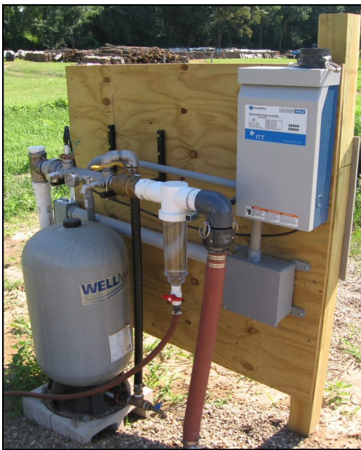
Submersible well pump controls.
