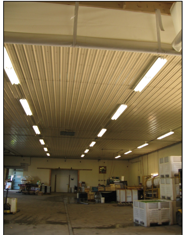
Overhead lighting was replaced with shorter, more efficient lamps.
