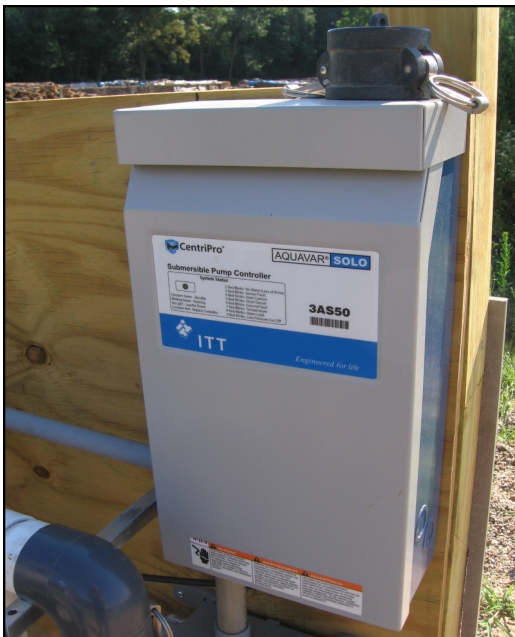
Close up of variable speed pump control.
