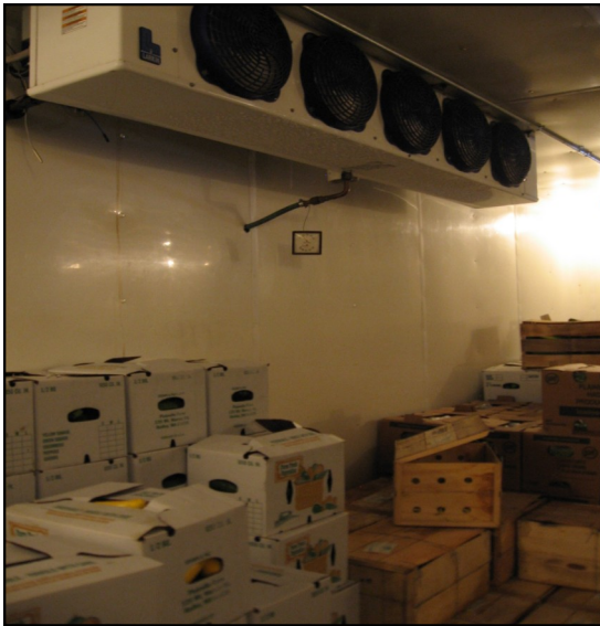
Cooler lighting and fan motor replacements.
