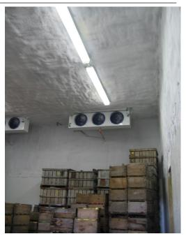
A variety of large and small refrigeration upgrades can help farms reduce energy. From left to right, high efficiency fan motors, outside air economizer, and an example of updated insulation and lighting.
