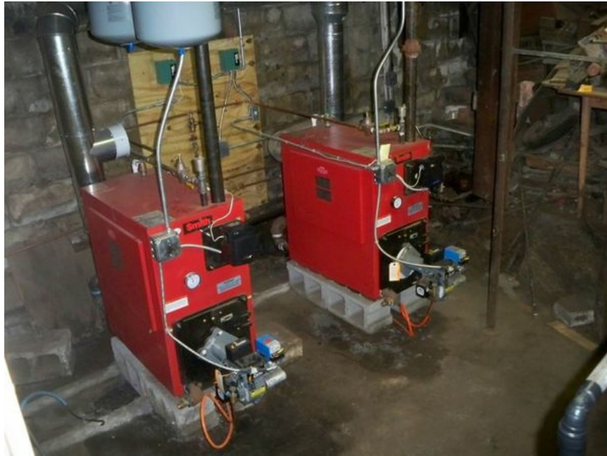
Efficient heater replacement at Dutchie's Greenhouse in Plymouth
