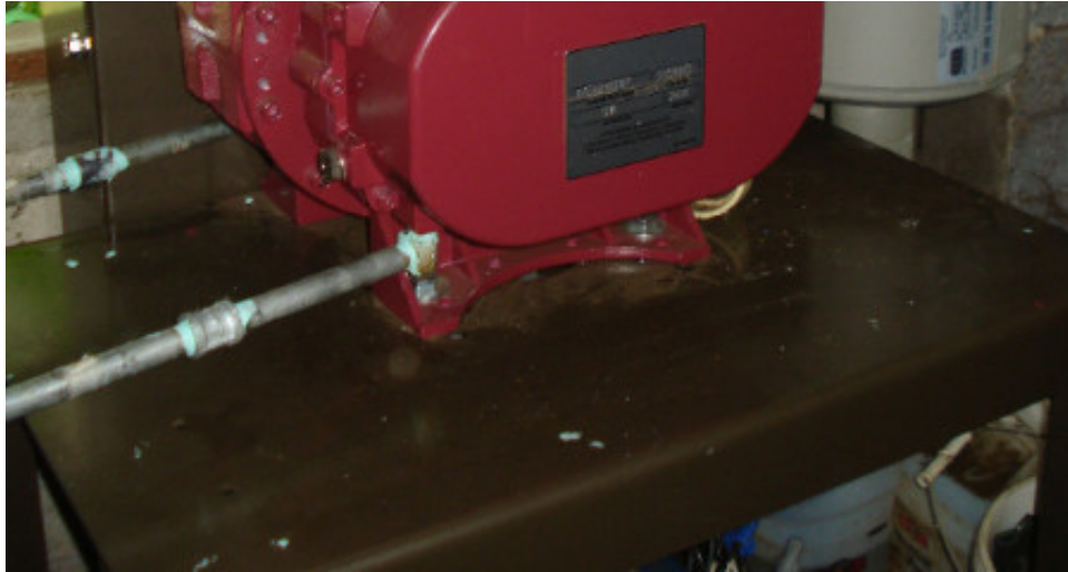
Example of a variable speed pump motor.
