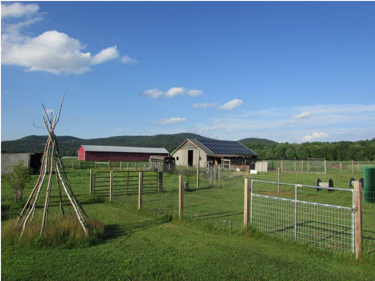
Roof mounted solar electric array at Little Brook Farm in Sunderland.
