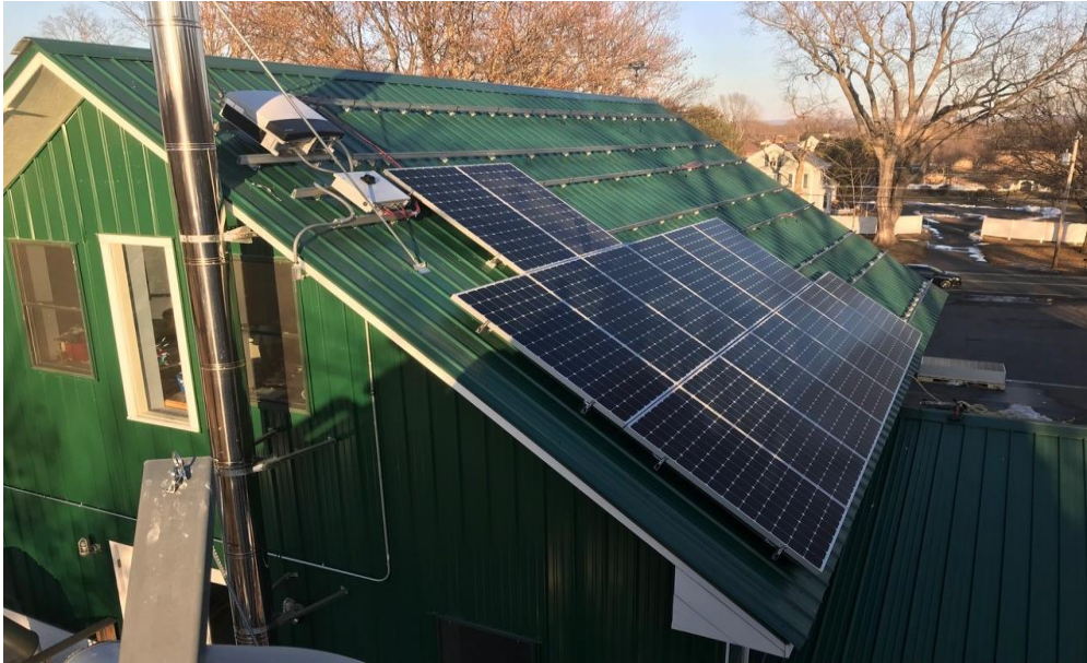
In-process roof mounted solar electric array at Valley Malt in Hadley
