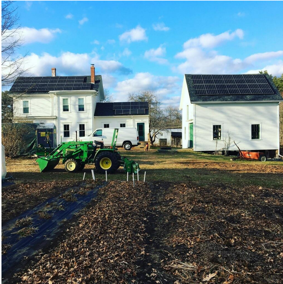
Roof mounted solar array at The Herb FARMacy in Salisbury
